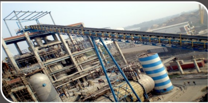
ERECTION OF FIBRE LINE EQUIPMENT
