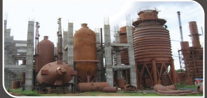
ERECTION OF DIGESTER & BLOW TANK
